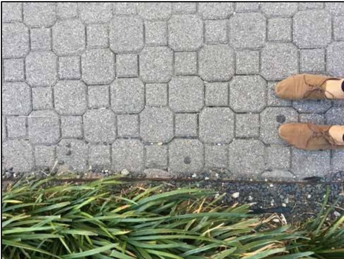
Figure 12. Permeable Pavement in Dallas, Texas<sup>165</sup>
